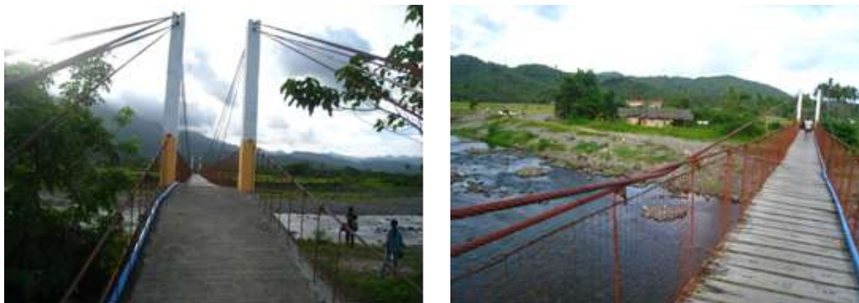
Figure 3.60 A hanging bridge was constructed by the provincial government to enable the farmers to cross the river
