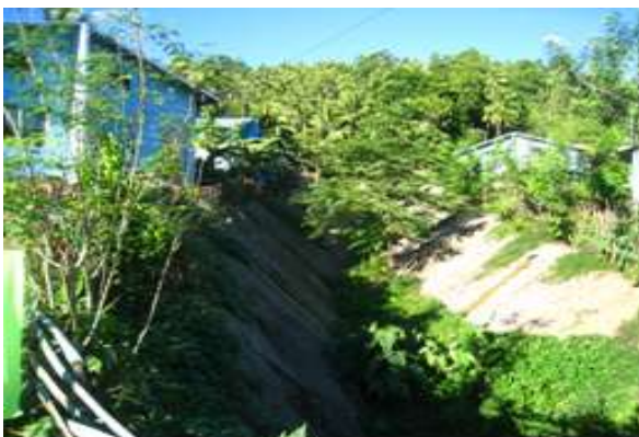
Figure 3.17 The paved embankments creeks (left) and natural embankments creeks facing the threat of hillside erosion
