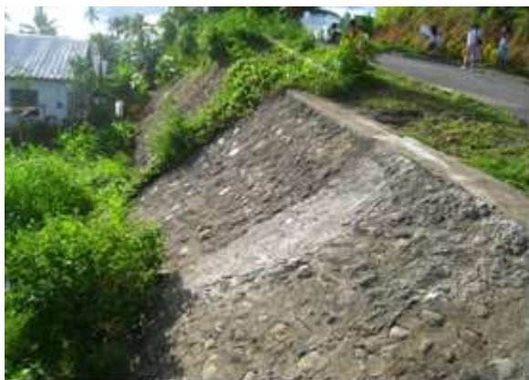
Figure 3.22 A road along the slope towards the village
