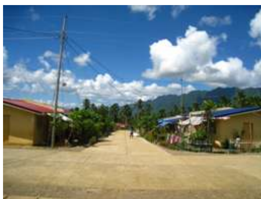
Figure 3.28 Cemented road within the resettlement
