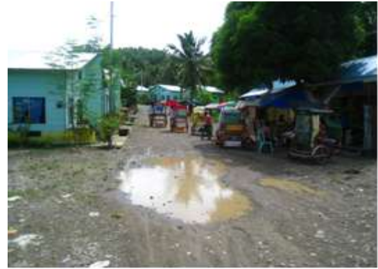
Figure 3.14 Condition of the road
