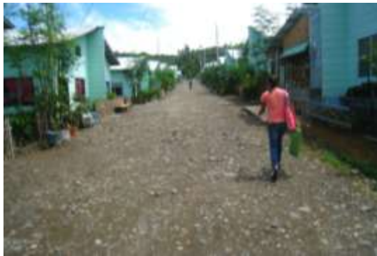
Figure 3.15 The road inside Ayahag resettlement
