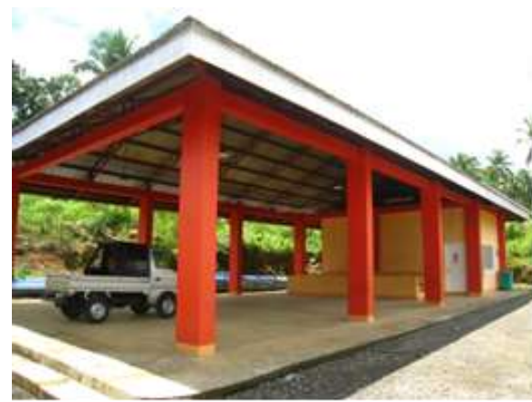
Figure 3.59 A multi-purpose covered hall in Mahika Resettlement
