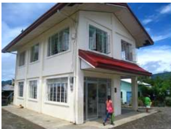
Figure 3.56 The building that houses the health center on the ground floor and the barangay hall on the second floor
