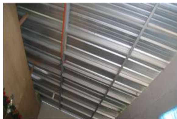
Figure 3.8 The hardiflex steel frame
