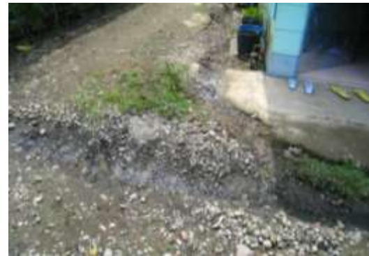
Figure 3.16 Surface drainage in Ayahag resettlement
