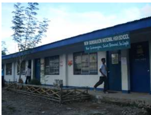
Figure 3.37 The structure of the New Guinsaugon High School
