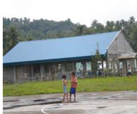
Figure 3.51 The chapel under construction
