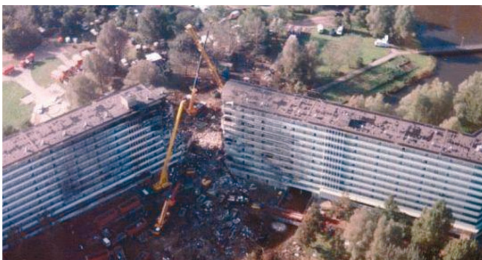
Figure 23: Apartment building after being hit by a Boeing 747 Amsterdam "Bijlmer", October 4th, 1992.
