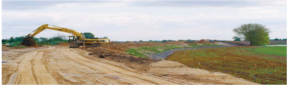
Figure 43 Widening and heightening of a dike
