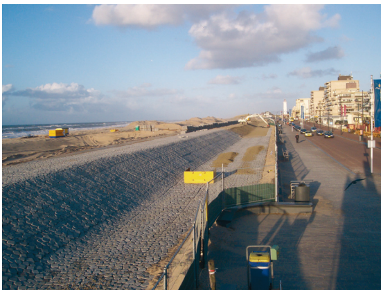
Figure 57: Coastal Flood Defenses in an Urban Environment, Noordwijk, Arcadis 2010
