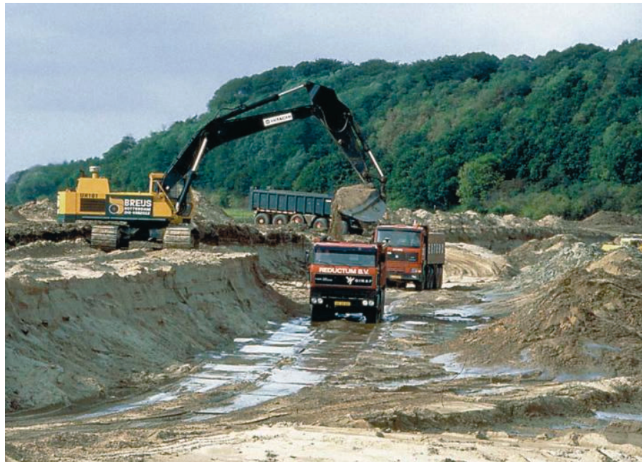
Figure 49: The construction of a side channel, “Blauwe Kamer Wageningen”
