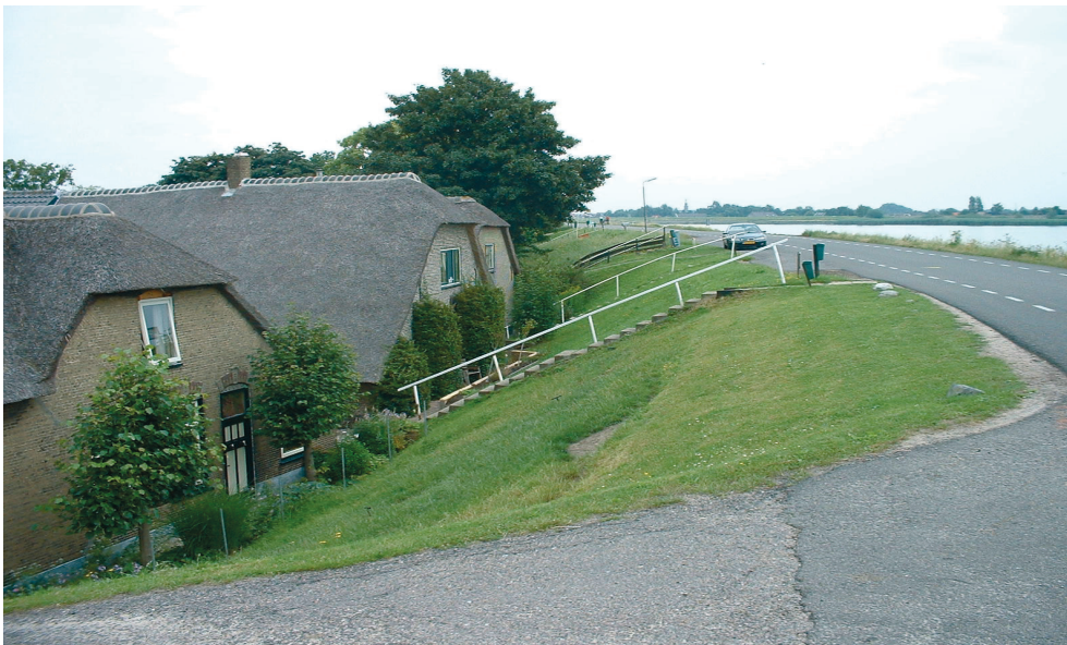
Figure 51: Houses built near the dike, after a number of dike reconstruction programs
