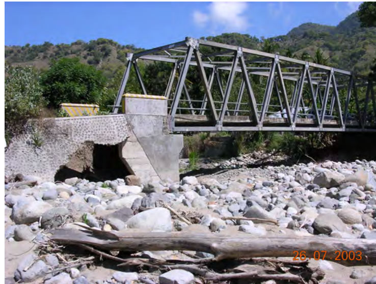
Schematic representation of a flashflood event (top) and image of a destroyed bridge foundation (left).
