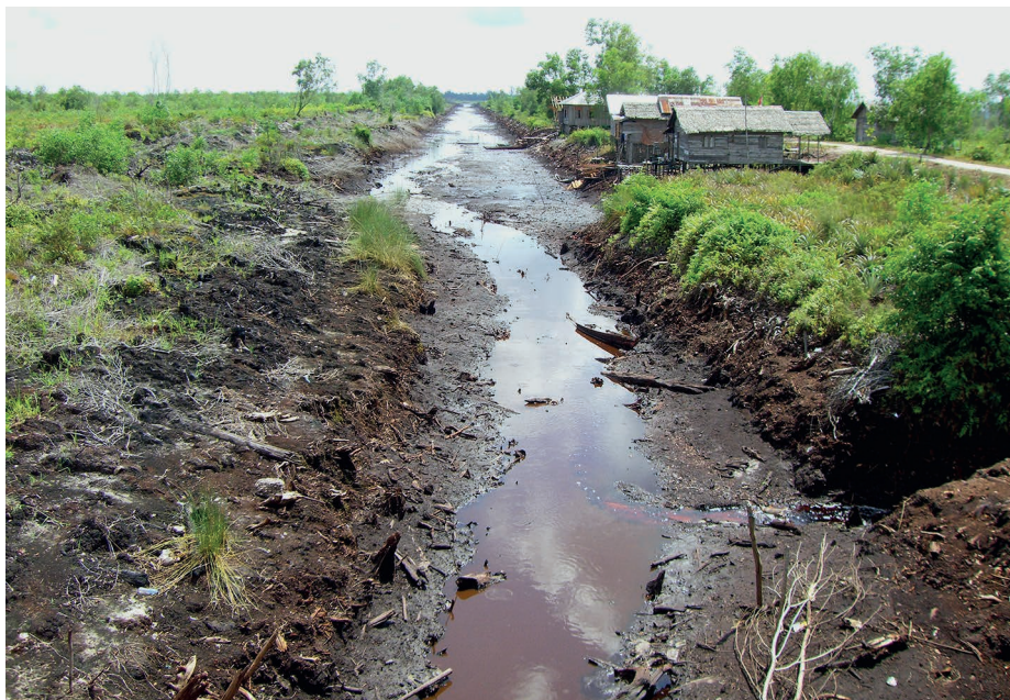
A canal on peatland. Canals such as this, located in the area of the former Mega Rice Project (Central Kalimantan province, Indonesia), were used to drain the peatlands. They will need to be dammed to re-flood the peat and rehabilitate it. © Luca Tacconi.
