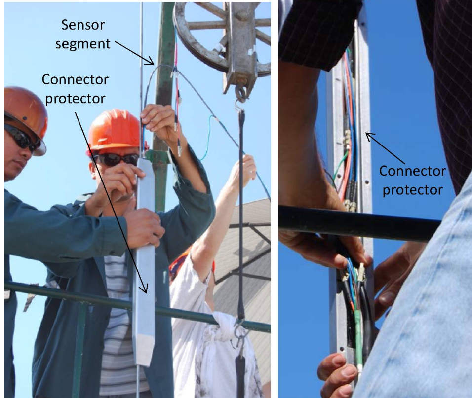
Figure 55 (left) Integration of the first connector protector and first sensor segment. (right) Optical connections inside the protector connector.
